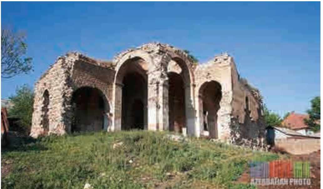
The church after its destruction—probably explosion—in the late 1990s (unknown photographer, 2003)
