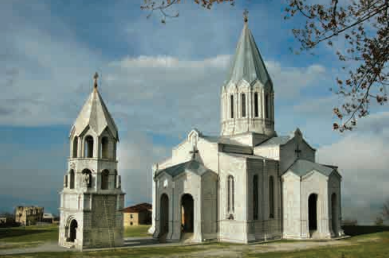
Sourb Amenaprkich (Holy Saviour) or Ghazanchetsots Church and its belfry after restoration (photo by S. Karapetian, 2008), Shushi City, Shushi District.
