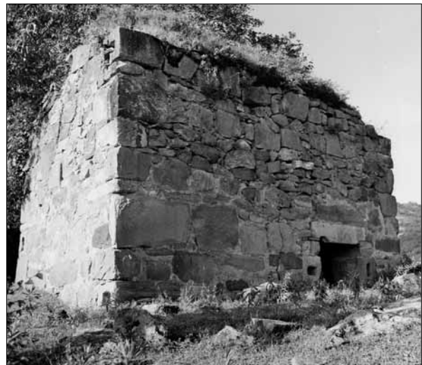
St. Sargis Church of Darpas Village from the north-east
