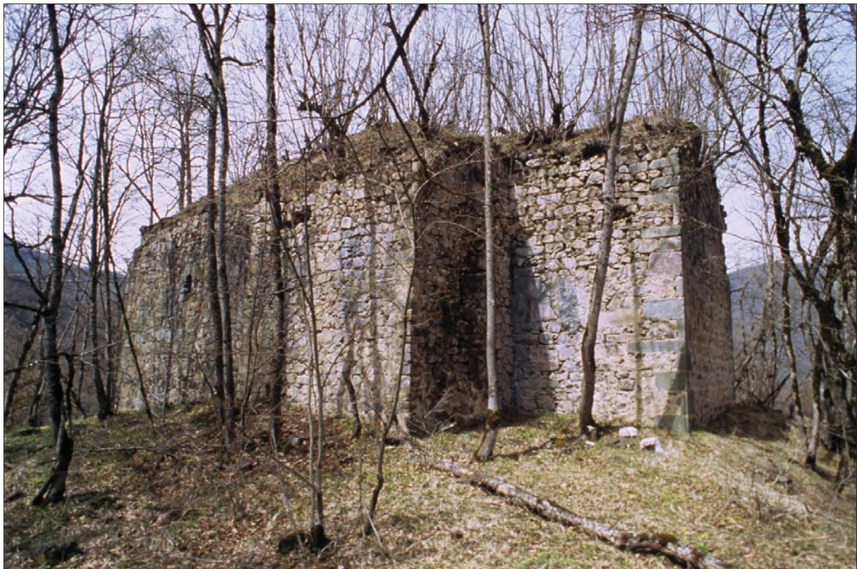
Khatravank as seen from the north-west and south-east (2011)
