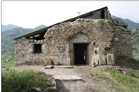
The southern part of the complex after the excavations
