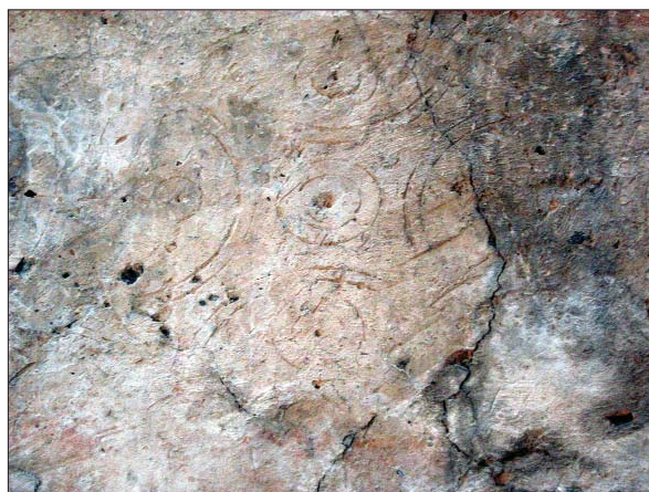
Ornament remnants on the plaster
