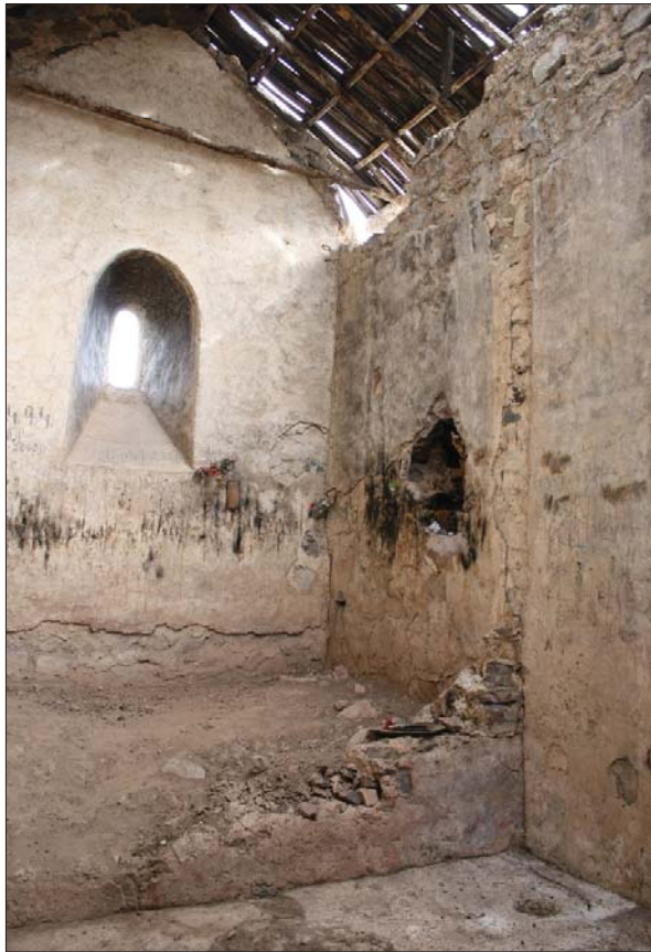
The church floor as flattened with mortar
