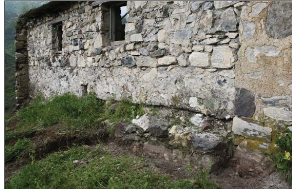
The unearthed thick retaining wall
