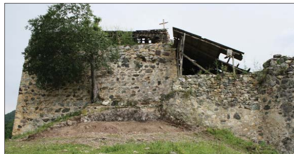
The remnants of a chapel unclosed north of the church
