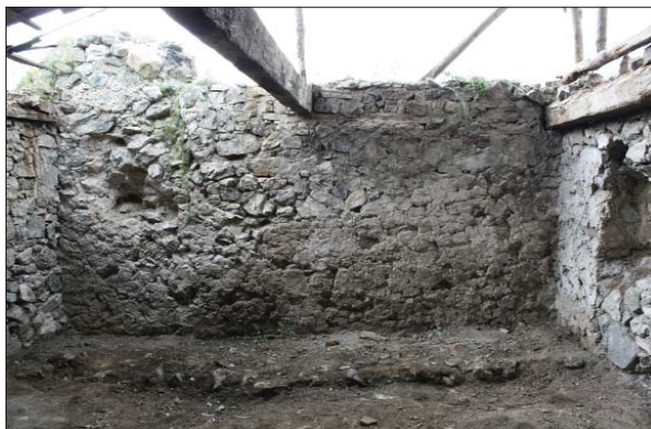
An inner view of the northern wall of the cattle house adjoining the church
