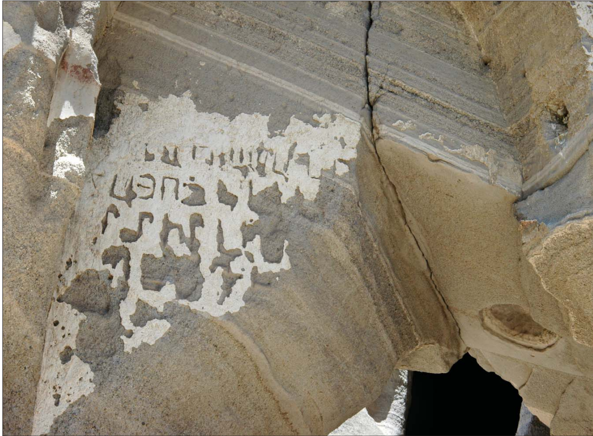
The remnants of an inscription (952), originally comprising at least four lines, preserved on the entrance tympanum of the porch adjoining the monastic church from the south
