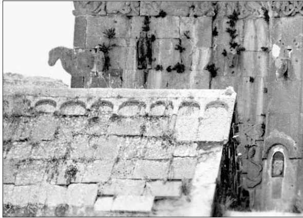
AGHTAMAR. The chapel located near the north-eastern corner of Sourb Khach Monastery: a partial view of its old indented covering slabs with cylindrical endings; the chapel roof after its revetment with smooth slabs
